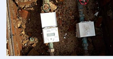
For the AMR (Automatic Meter Reading) on Kaprije, the existing mechanical water meters were successively replaced by static HYDRUS ultrasonic meters. For the radio readout, two unidirectional antennas were installed and the IZAR RDC Premium Receiver is configured to upload the meters data every 15 minutes to the Diehl Metering FTP server. The data management system is provided by the local partner company IKOM.
